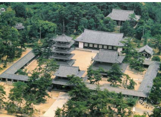
Left: A grove of cypress trees prepared for harvest. Above, left: Built in 607, Horyuji monastery is Japan's oldest surviving example of monumental timber-frame architecture. Its five-story pagoda (top) enshrines relics of the Buddha. The pagoda's main structural element, pictured in the cutaway (right), is its heart pillar, a single cypress tree that keeps the building steady during earthquakes. Above, right: More cypress pillars hold up the monastery's outer ring and main hall.
